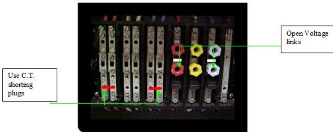
Figure 11 Shorting out CTs and opening voltages for white phase load test
