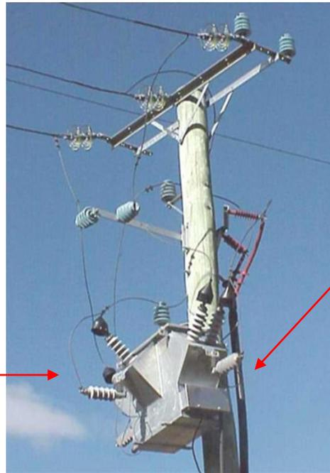
Normally installed so that phase sequence is in the standard A, B, C configuration
