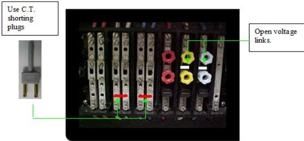
Figure 10 Shorting out CTs and opening voltages for red phase load test
