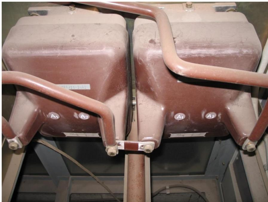
Figure 30 Siemens 22 kV to 110 V transformer
