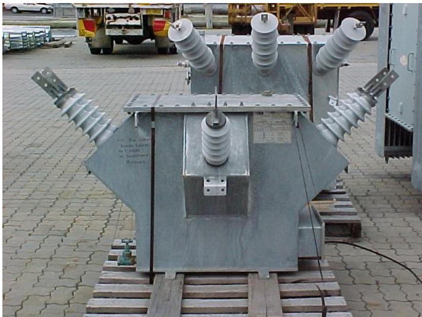
Figure 16 ABB pole-mounted HV metering unit
