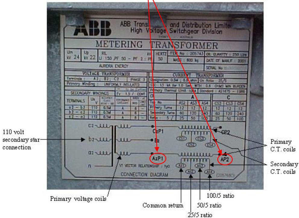
Figure 21 Terminals and wiring diagram showing matching numbers of an ABB metering unit
