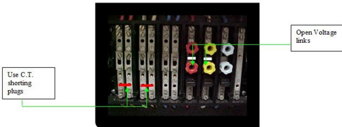
Figure 12 Shorting out CTs and opening voltages for blue phase load test
