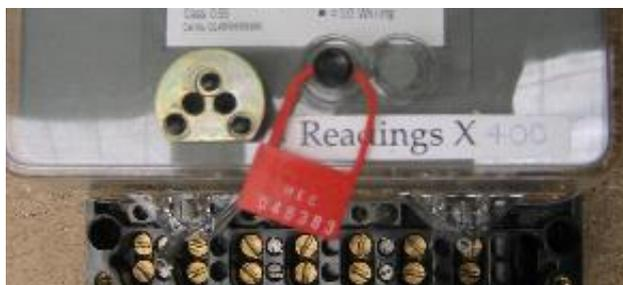
Isolation switches can be sealed in the off position using a non-renewable plastic seal type. The product details of this approved seal is PULL SECURE EN4011. Note that this seal must not be used for any other purpose.
