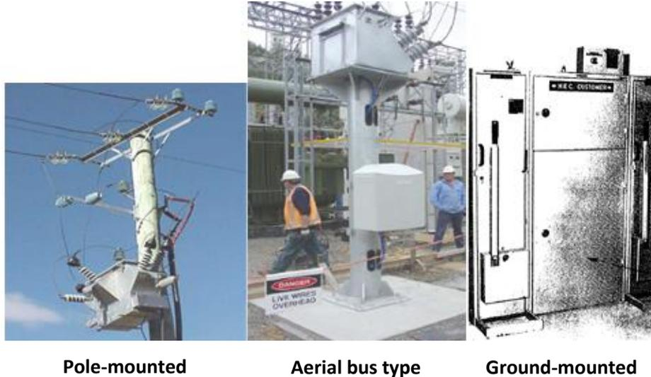
Figure 13 HV metering installation types
