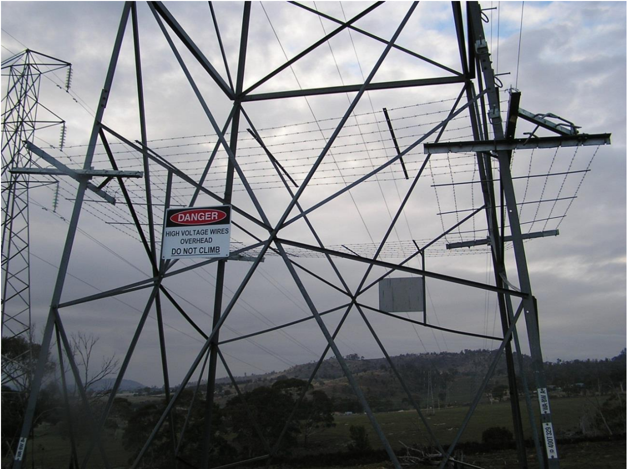
Figure 1 – Standard climbing barrier general arrangement
