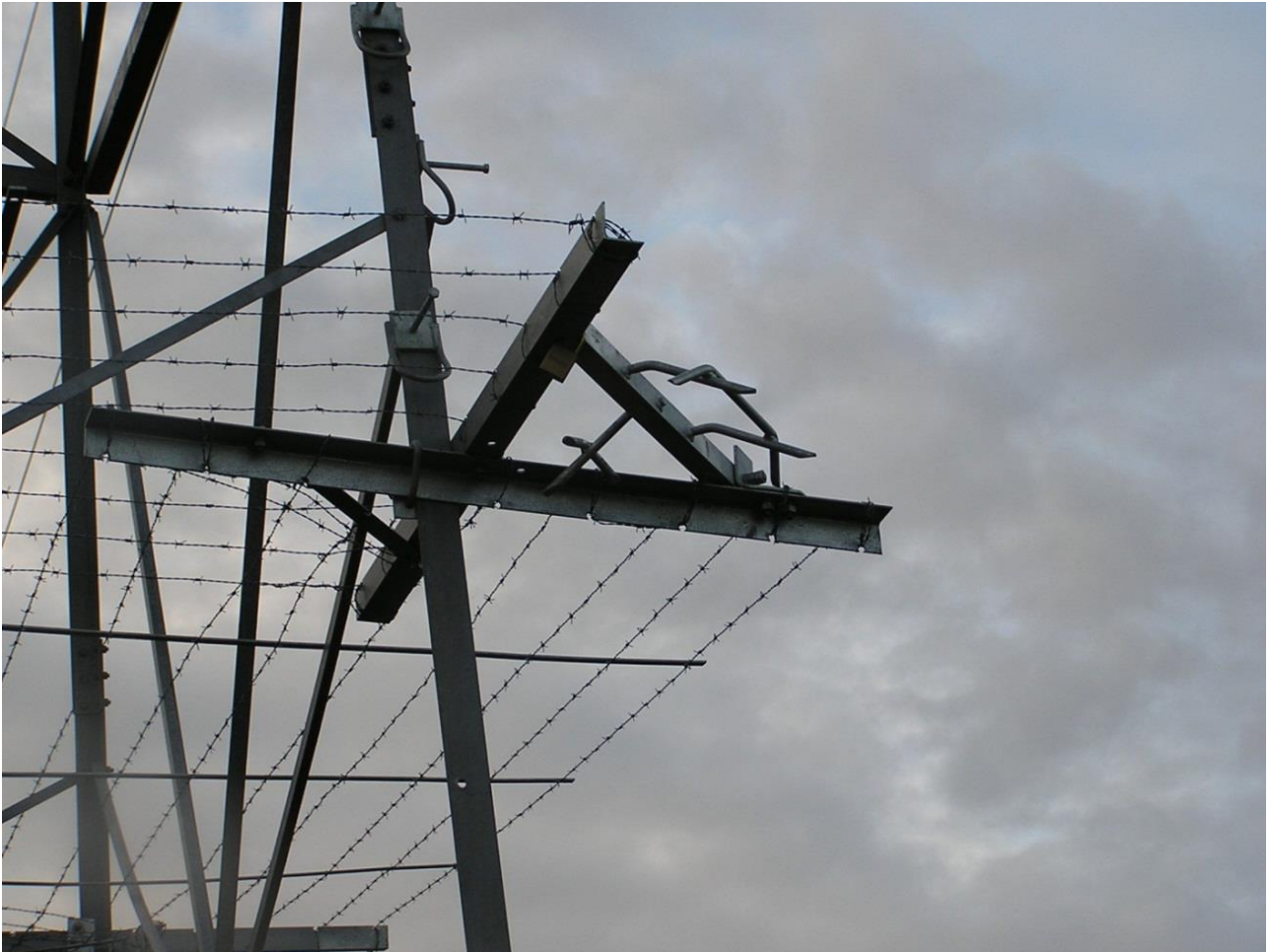
Figure 2 – Standard climbing barrier corner arrangement
