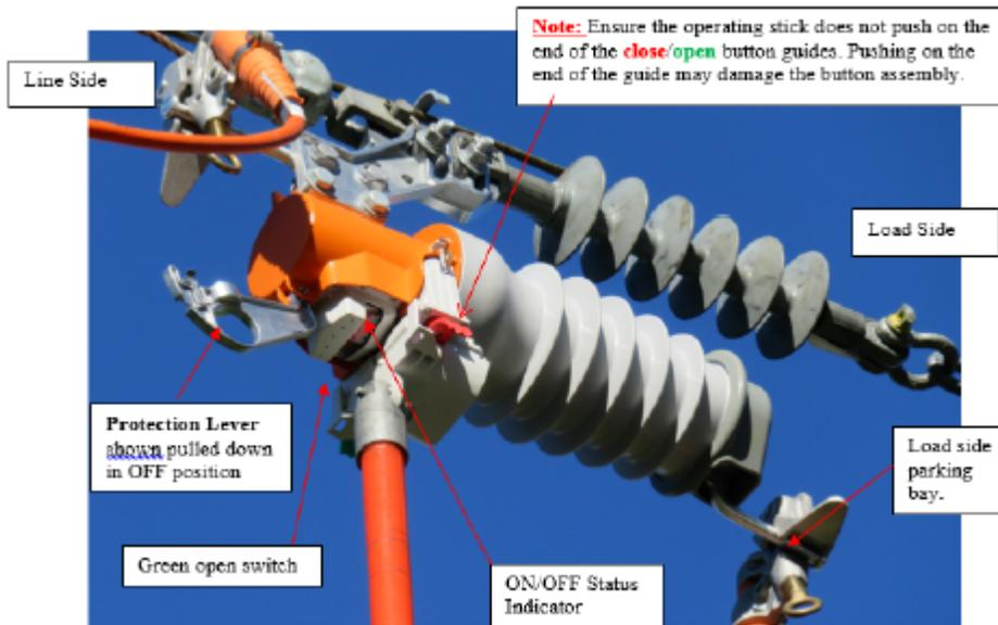
Fig. 3 Isolation Switch With Battery Pack & Comms. Module Inserted And Protection Lever Pulled Down Into Off Position
