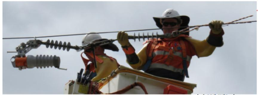
**NOTE:** Bridging leads connected prior to operating the switches.
