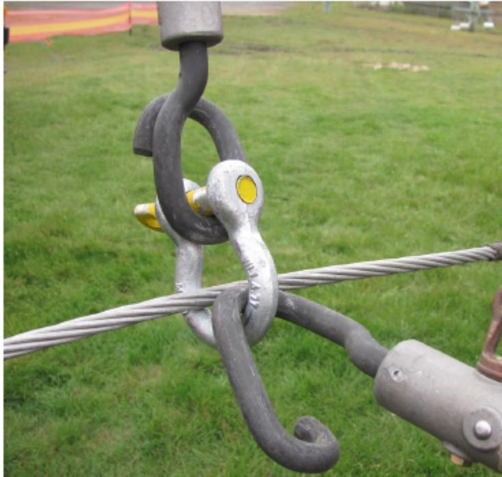
11. Take weight on side ropes utilising rope blocks. These are to be secured to a vehicle.
