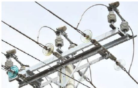
Older type air break switch
