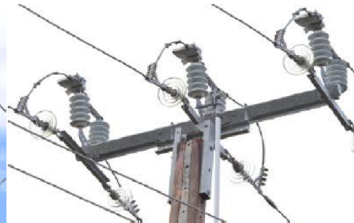
Stanger, USB air break switch
