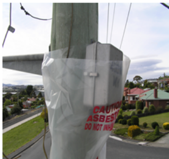
Remove lower bolt and slide Approved bag up over Choke Box
