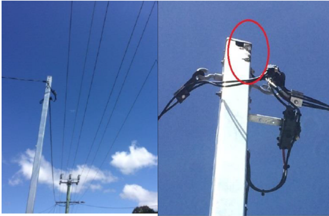
Pole too close to Overhead HV Result – arcing and broken conductor
