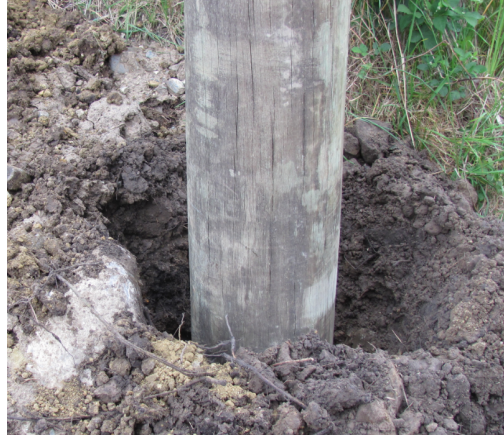
Typical Pole Hole Dug Out.
