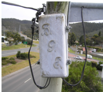
GEC Hinged Type Choke Box Asbestos Seal and PCB Capacitor
