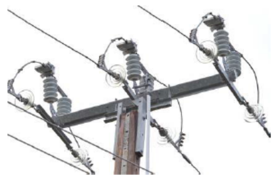
Stanger, USB air break switch
