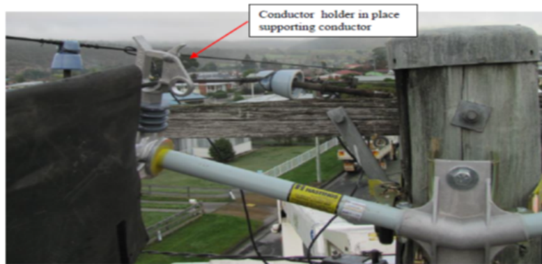
Example Of V Type Temporary Cross Arm Being Used
