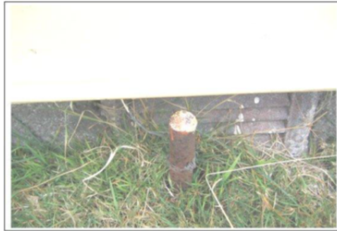
Example of poor earth connection
