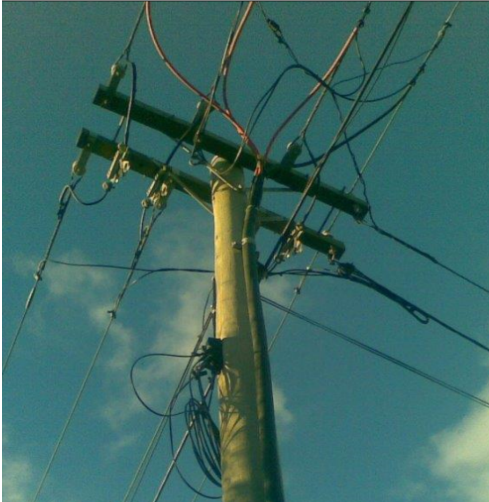
Example Standard LV Underground Cable Termination On Pole
