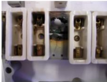
Failed active bus on federal switchboard
