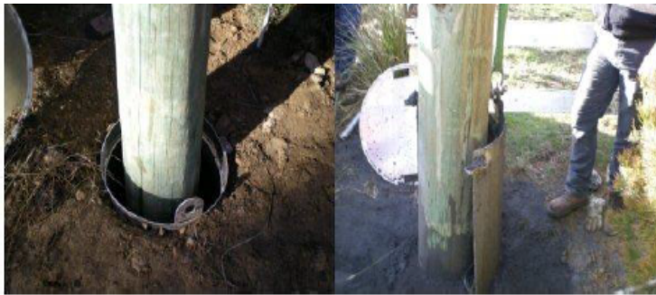
Cover removed – while pole held steady.
