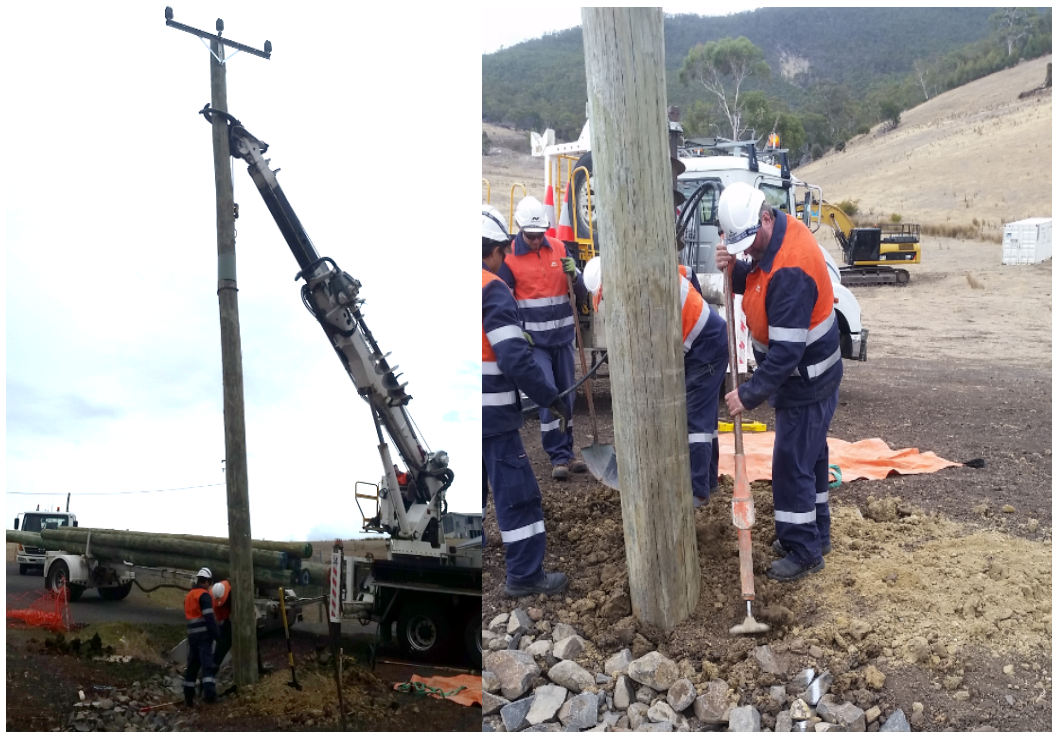
Check clearances before backfilling Solid ramming and tamping
