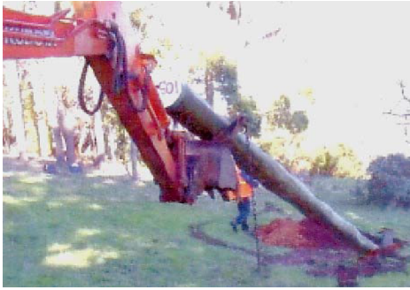
Push Method Using Supporting Jig
