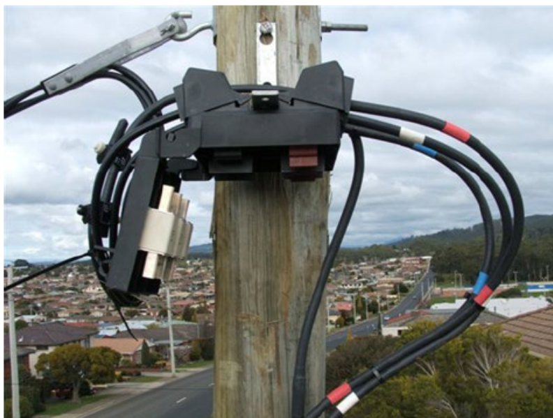
Example of Three Phase UG Cable Termination On Pole
