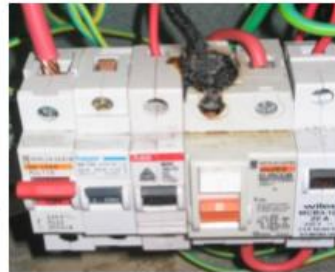
Loose RCD connection
