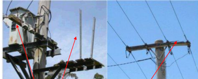
Suspect cross arm end & broken platform rail
