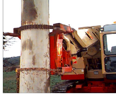
Lift Method Using Pole Grab
