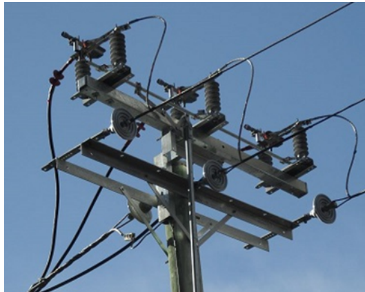
Typical Air Break Switch
