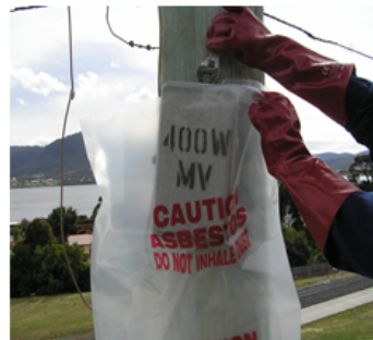
Remove upper bolt and lower Choke Box into Approved bag
