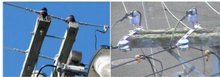
Cross arm end split – loose insulator pin Old rotten cross arm moss covered.
