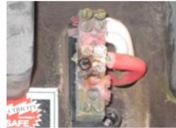
Poor termination / corrosion on link
