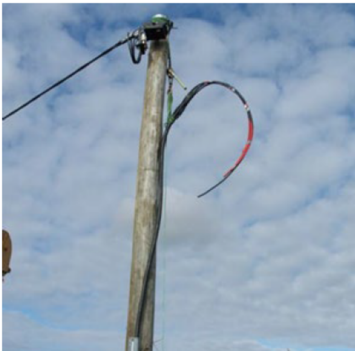
Example of UG Cable Being Tensioned Up Ready For Connection
