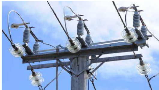
ABB, S Series air break switch
