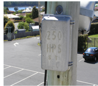
AEI Hinged Type Choke Boxes Asbestos Seal and PCB Capacitor
