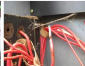
Termination loose - over heating
