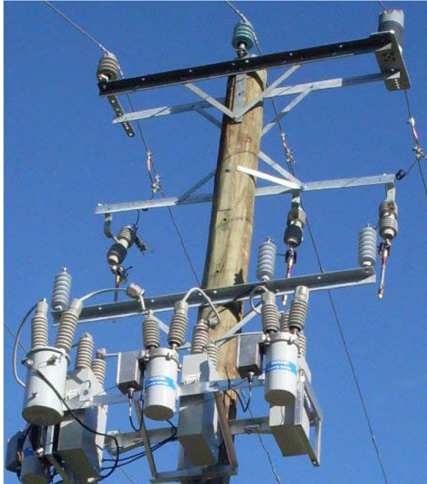
Typical Capacitor Bank Installed
