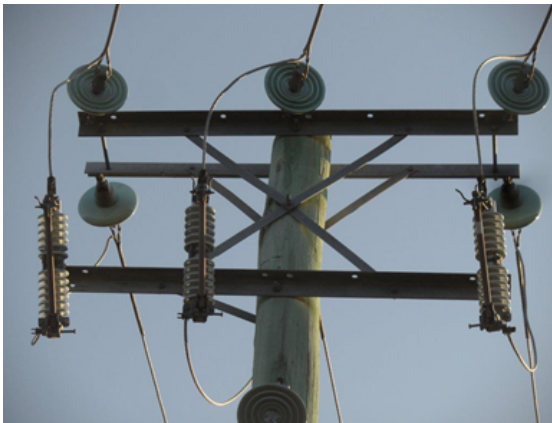
Typical EDO Fuse Switch
