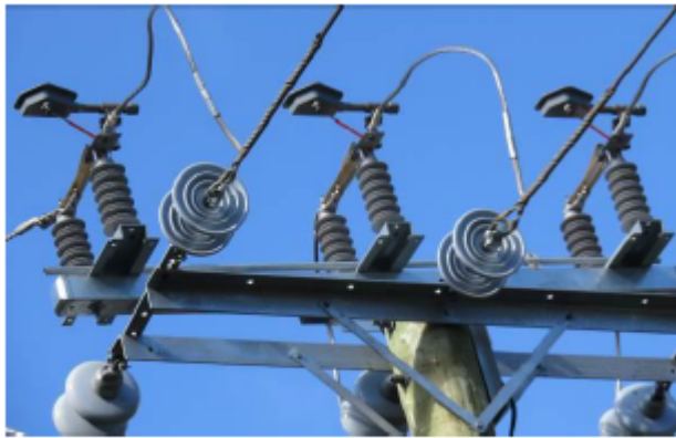
Figure 1: Typical AK Power air break switch
