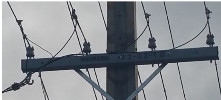
MK1 Fibreglass cross arm installed on a stobie pole
