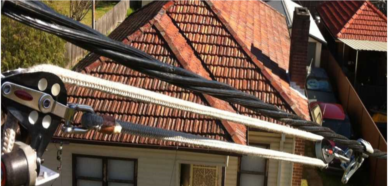
Typical cable strain grip and comealong on ABC service
