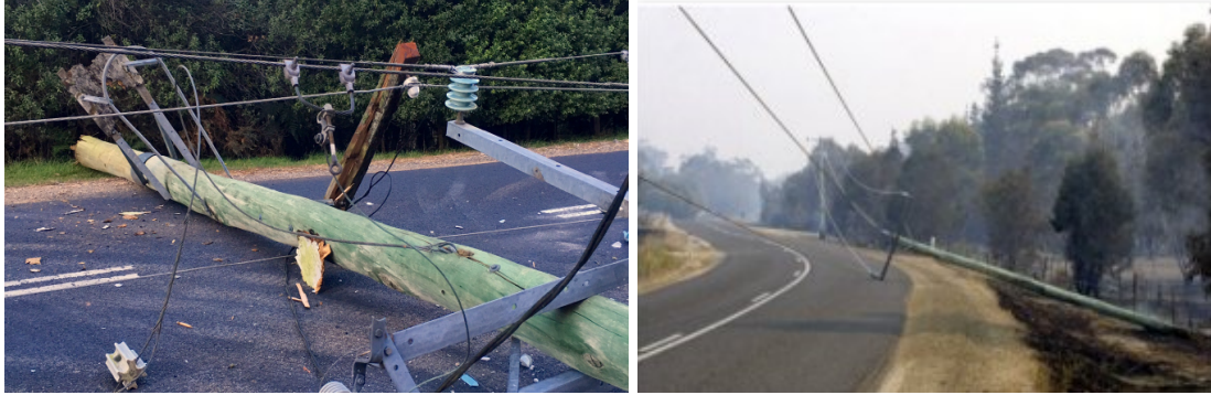
Examples of fallen poles – caused by bush fire or storms.
