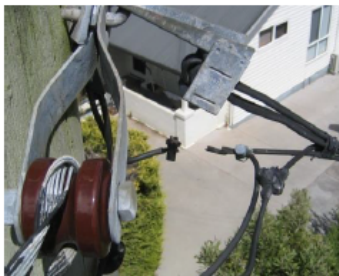
Broken service neutral at pole
