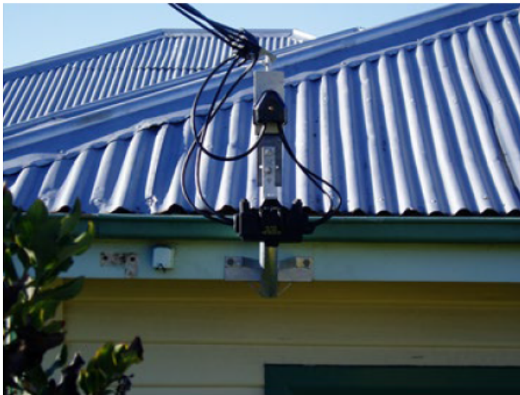
No drip loops and, no cable ties used.
