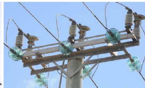
Morlynn/Stanger air break switch
