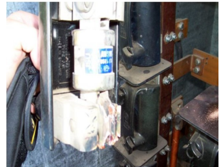
Example of damage caused reclosing onto a fault or large load
