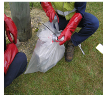
Secure with cable tie, fold over excess part of bag and secure with duct tape.
