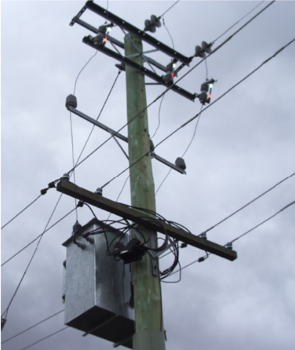
Typical Standard Three Phase Pole Mounted Transformer
