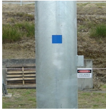
Figure 1 Example of blue phase identifier on an incoming circuit
