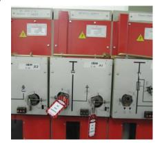
Each distribution switchgear key must be uniquely numbered to reference the owner on the key register.
